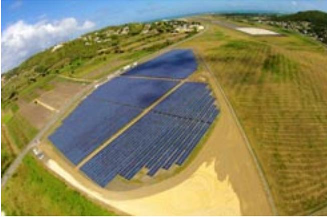
In 2016, Antigua installed this 3-MW ground-mounted solar power plant project at its newly constructed V.C. Bird International Airport. This was Antigua's first major infrastructure project to utilize renewable technology.
